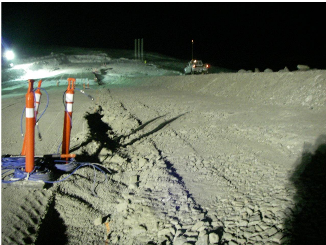
Photo 11: Transition material was placed and compacted along the downstream side of the frozen core. Photo looking south from Sta. 1+75
