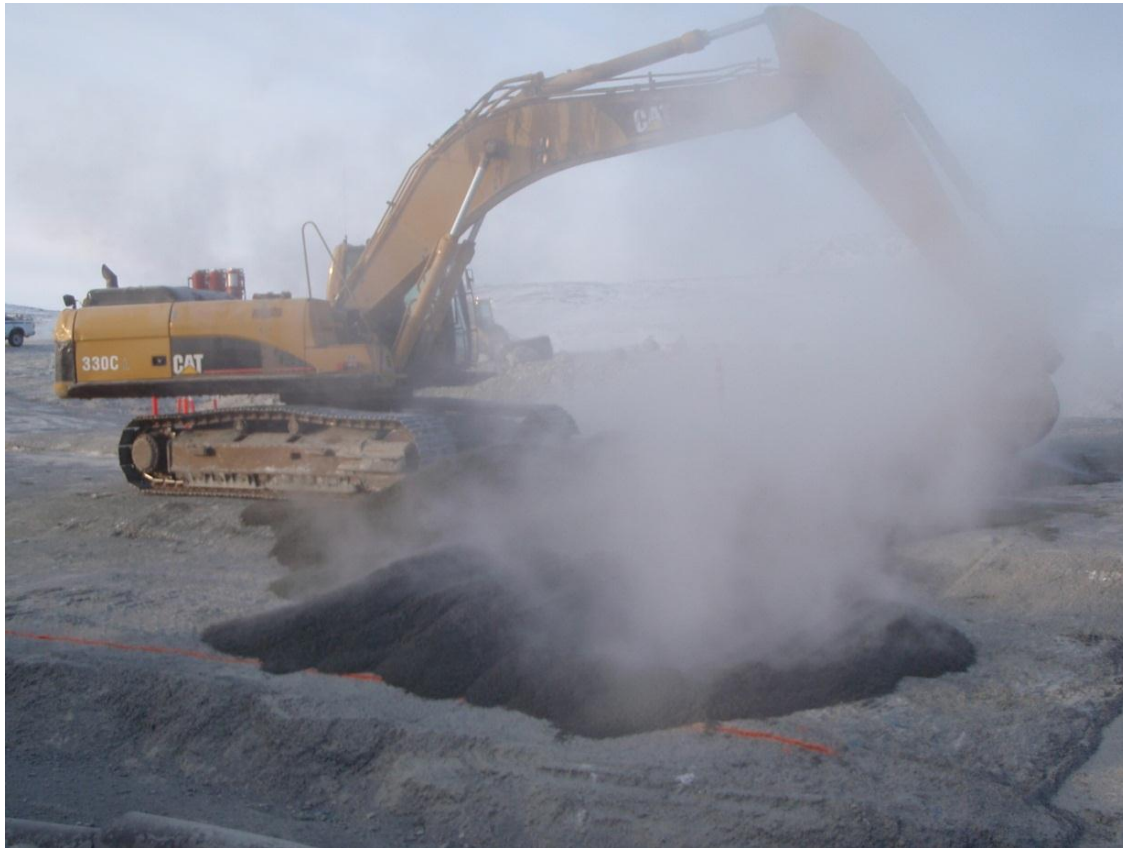
Photo 4: Cat 330 excavator spreading the first load of today's FCM.
