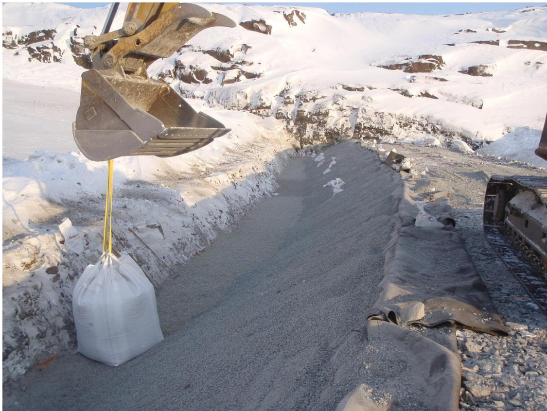
Photo 7: Excavator lowering bentonite chip mega-bags into the base of the key-trench
