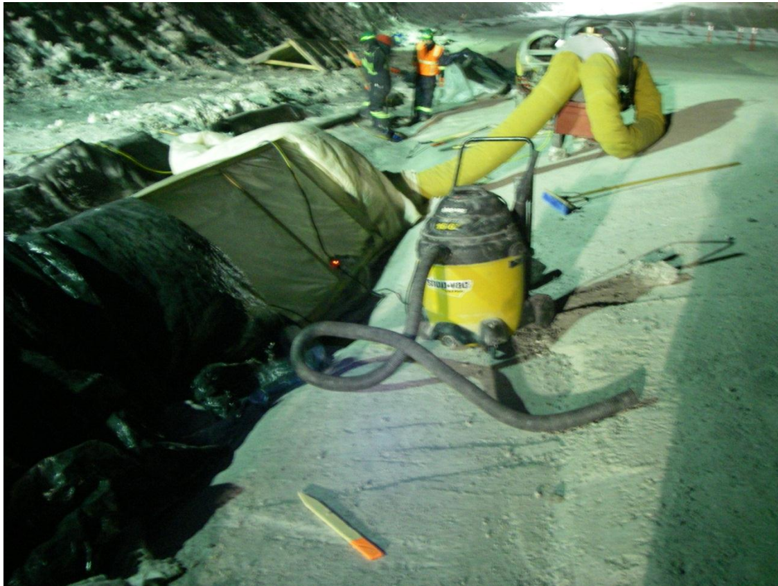
Photo 10: A Shop-Vac was set up to remove the meltwater before re-freezing.
