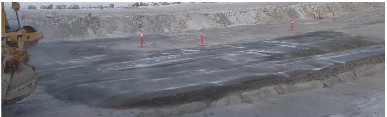
Photo 5: Photo during core placement today (foreground) was similar to placement yesterday (background, under delineators). This photo illustrates, to some degree, the appearance of the new FCM during placement and after freeze back.
