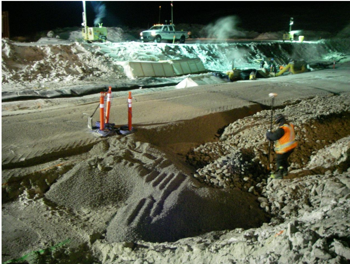
Photo 8: Thermistor cables at Sta. 1+75 were encased in dry core material. Surveyor picking up the extent of the transition material placement on the right side of the photo.
