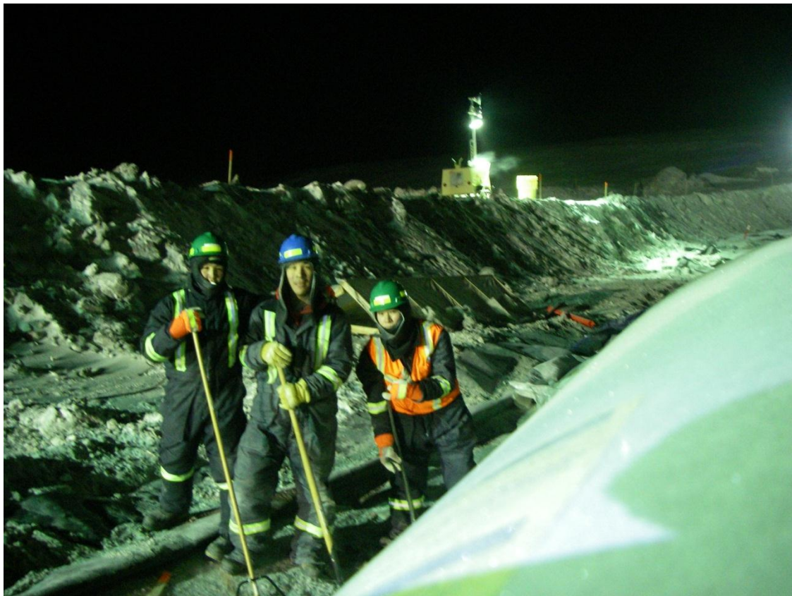
Photo 9: Workers hand cleaning the ice from the upstream edge of the keytrench.
